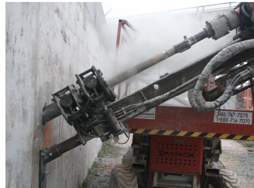
Installing retaining wall anchors
