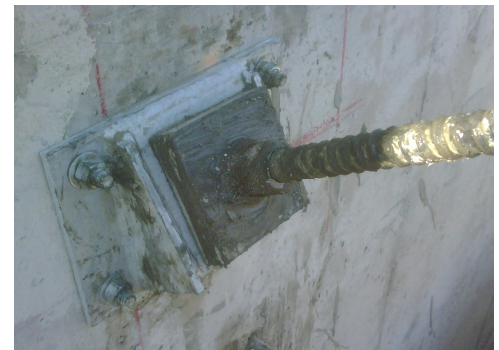
Termination at retaining wall
