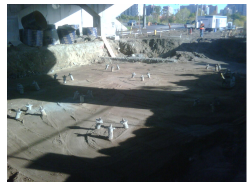
Installed micropile groups for new structure
