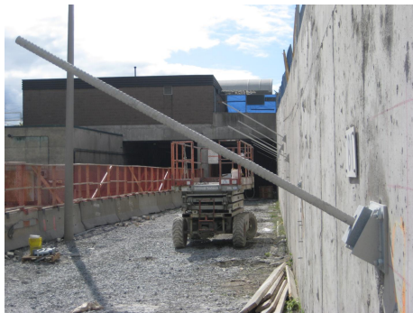
Micropile anchors installed along wall
