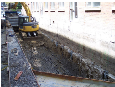
Piers installed – excavation beginning
