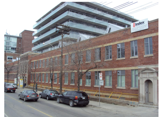
Warehouse structure before renovations
