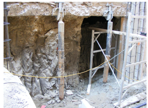
Sleeved helical piers during excavation operations
