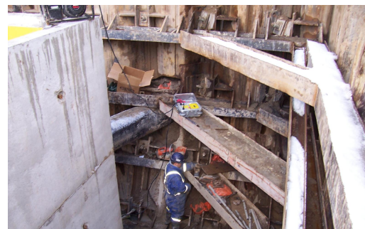
Installation of manhole within retained area
