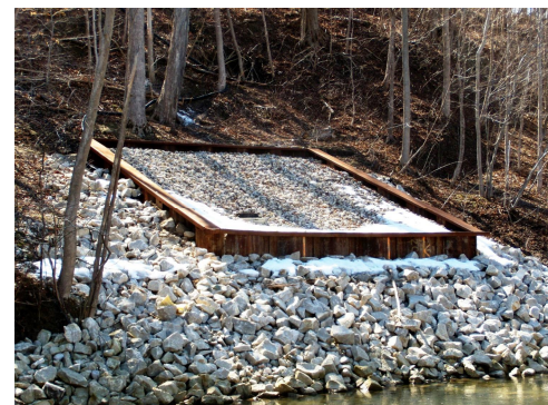
Completed backfilled area after construction
