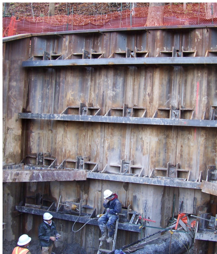
Completing fourth of five rows of anchors
