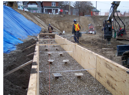
Grade beam forming before reinforcing steel added
