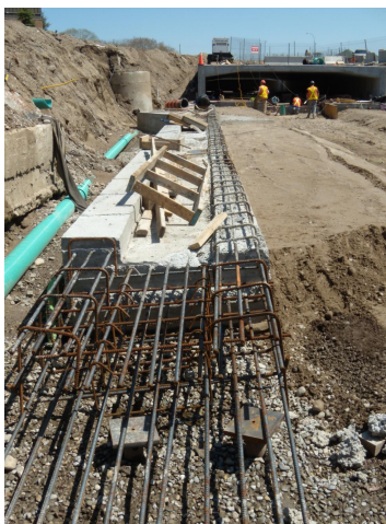
Installed piers cast in grade beam
