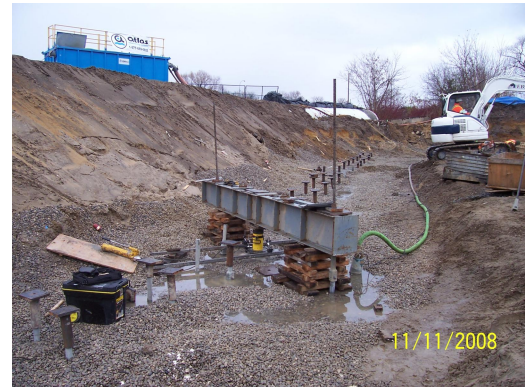
Load test being completed on a production pier
