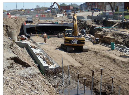
Overview of working area and culvert structure
