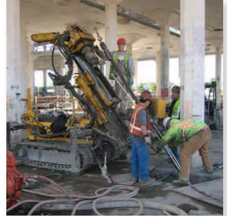
Figure 2: Battered micropile installation in an existing structure
