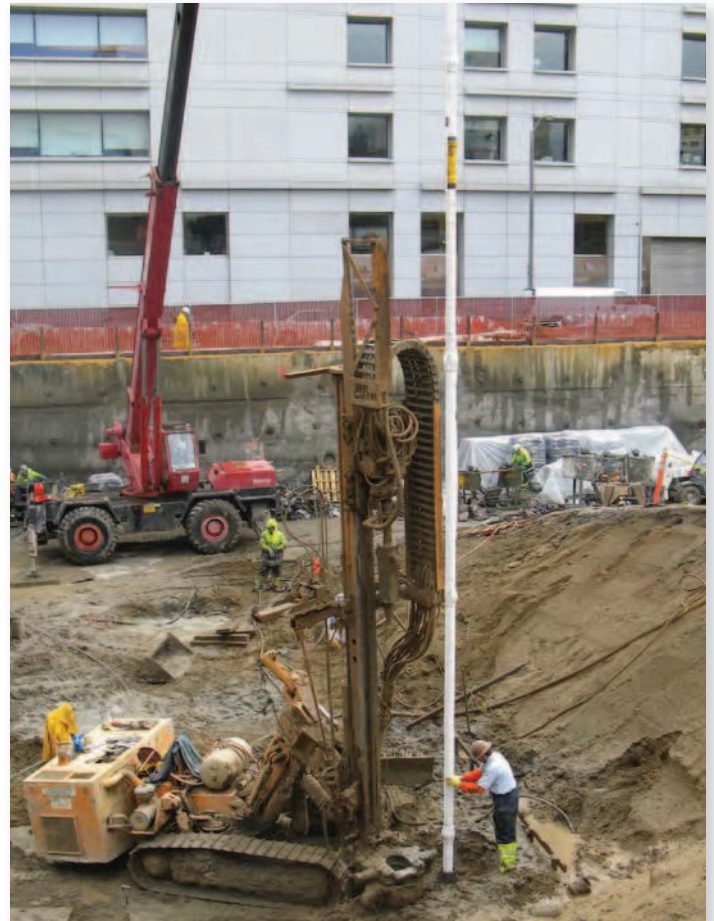
Figure 15: Micropile installation
