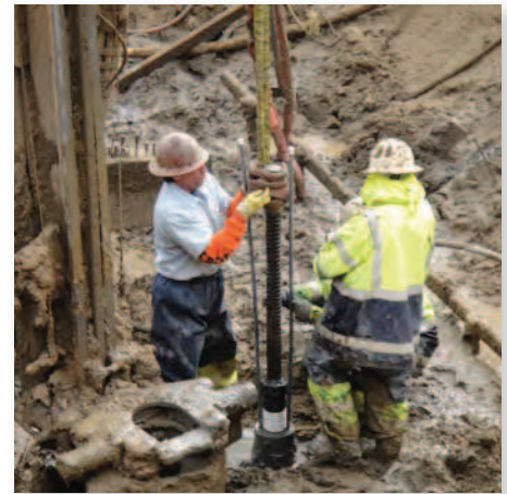
Figure 12: Installation of postgrouted micropiles
