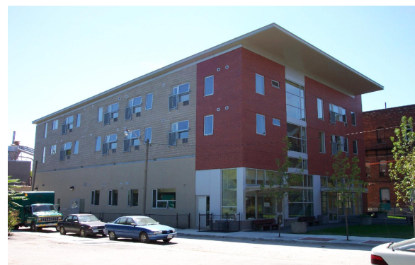
Finished structure with two additional storeys
