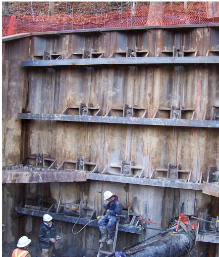
Completing fourth of five rows of anchors
