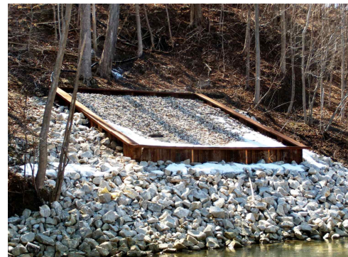
Completed backfilled area after construction
