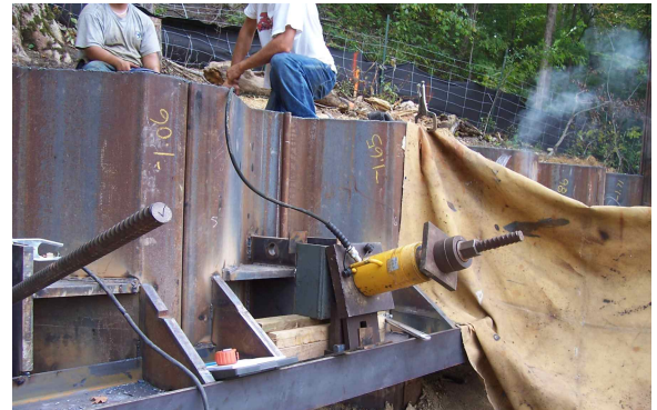
Proof loading of anchors to 133% design and locked off at 100% design load
