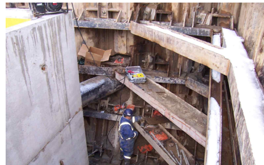
Installation of manhole within retained area
